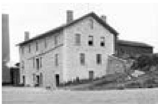
Brine Pump House in Syracuse
